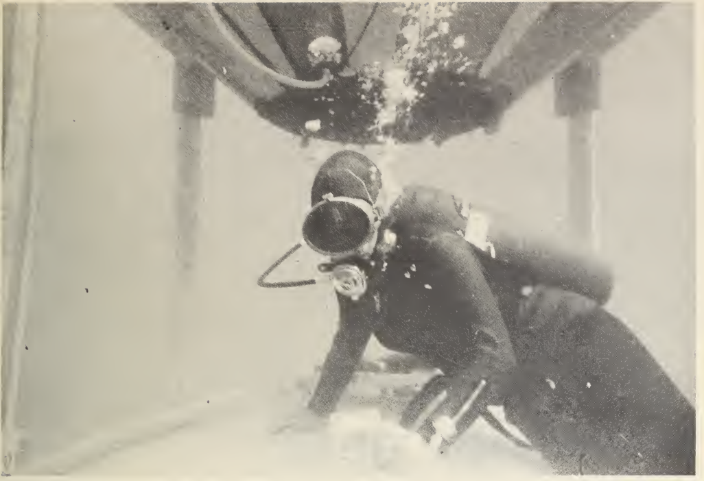
Sublimnos is entered through a vertical and completely open hatchway, visible behind and above the diver. A diver removes his aqualungs outside, hangs them on the exterior wall, and swims six feet to the hatchway, holding his breath.
